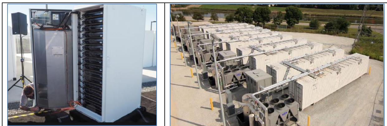
Figure 5: Solid state battery module (left) and system (right) Sources: Engadget.com
