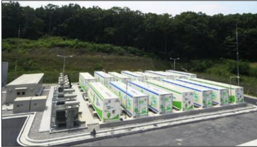
Figure 2-15: Example of a Lithium-Ion BESS installation
