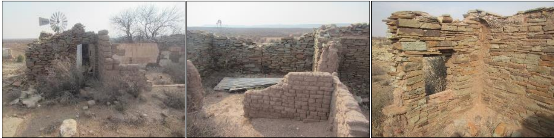
Figure 7-84: Part of a house at waypoint 112 in HL02 (left) showing sun-dried bricks, stone walls and a filled in doorway (middle) and showing stone walling and a remnant of a brakdak
