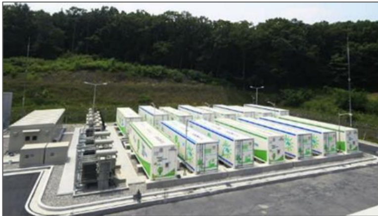
Figure 2-15: Example of a Lithium-Ion BESS installation
