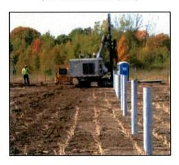
Figure 7: Driven/Rammed Steel Pile
