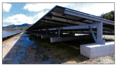
Figure 6: Cast Concrete Foundation
