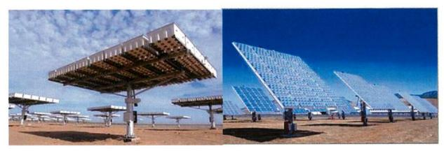
Figure 10: Loose-standing CPV modules.
