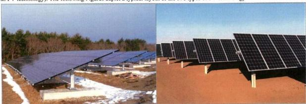
Figure 9: Examples of PV module arrays: flxed-tllt system (left) and single-axis tracking system (right).
