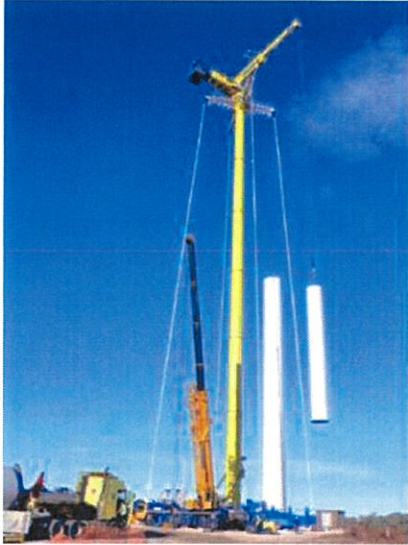
Figure 6: Example of cranes at work to erect the single turbine at Coega in the Eastern Cape
